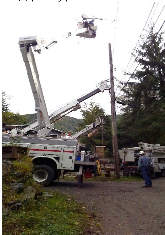
Collins Road Primary Work – “Cut and Kick” pole replacement
